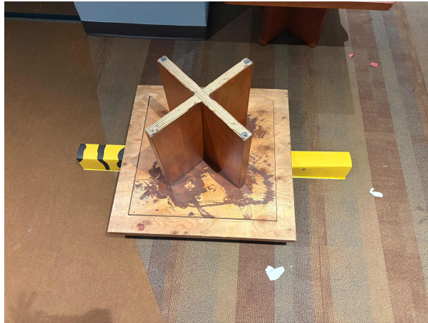
Figure 12: Weight on beam to ensure secure connection, Nov 22, 2025 1:08AM
